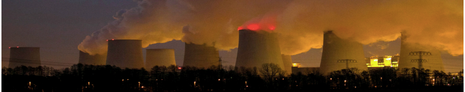
Cooling towers at the lignite coal-fired power plant in Janschwalde, Germany. Photographer: Krisztian Bocsi/Bloomberg
