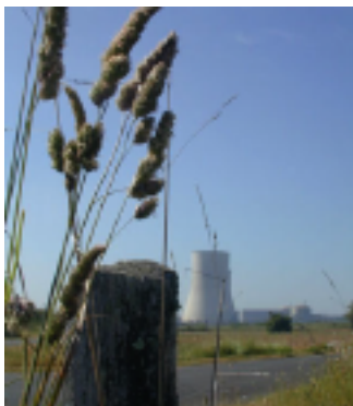
The Civaux Nuclear Power Plant
