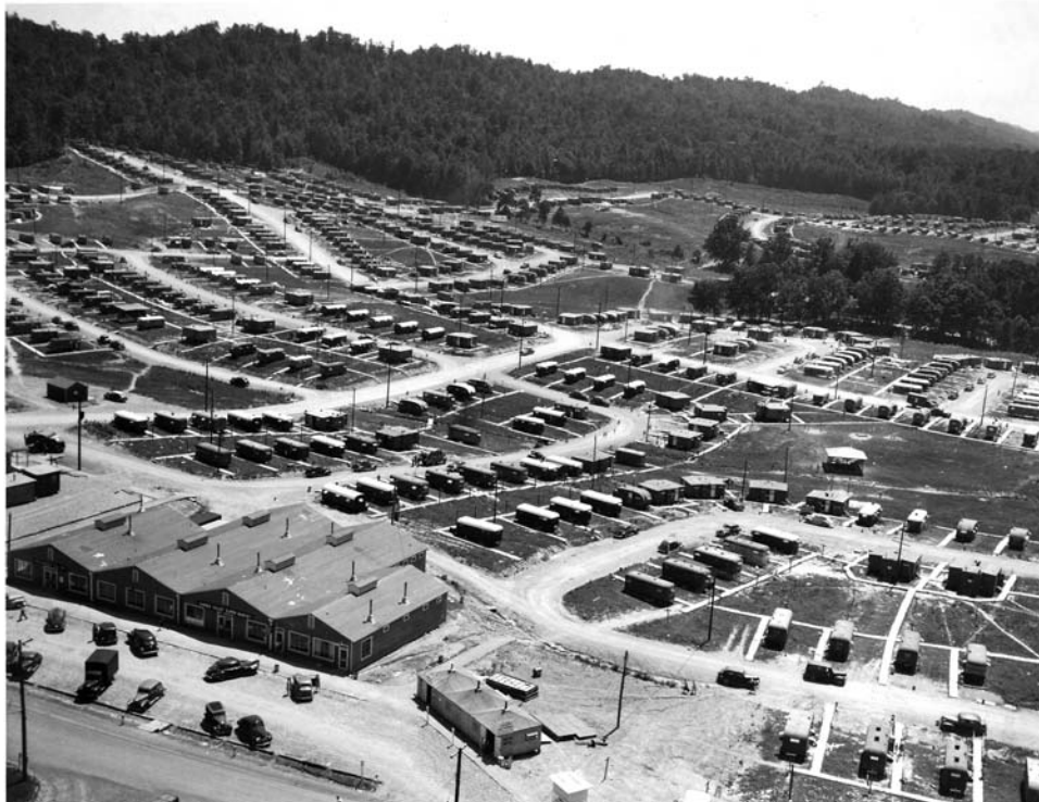
Figure 2.4 Construction camp trailers (DOE)
