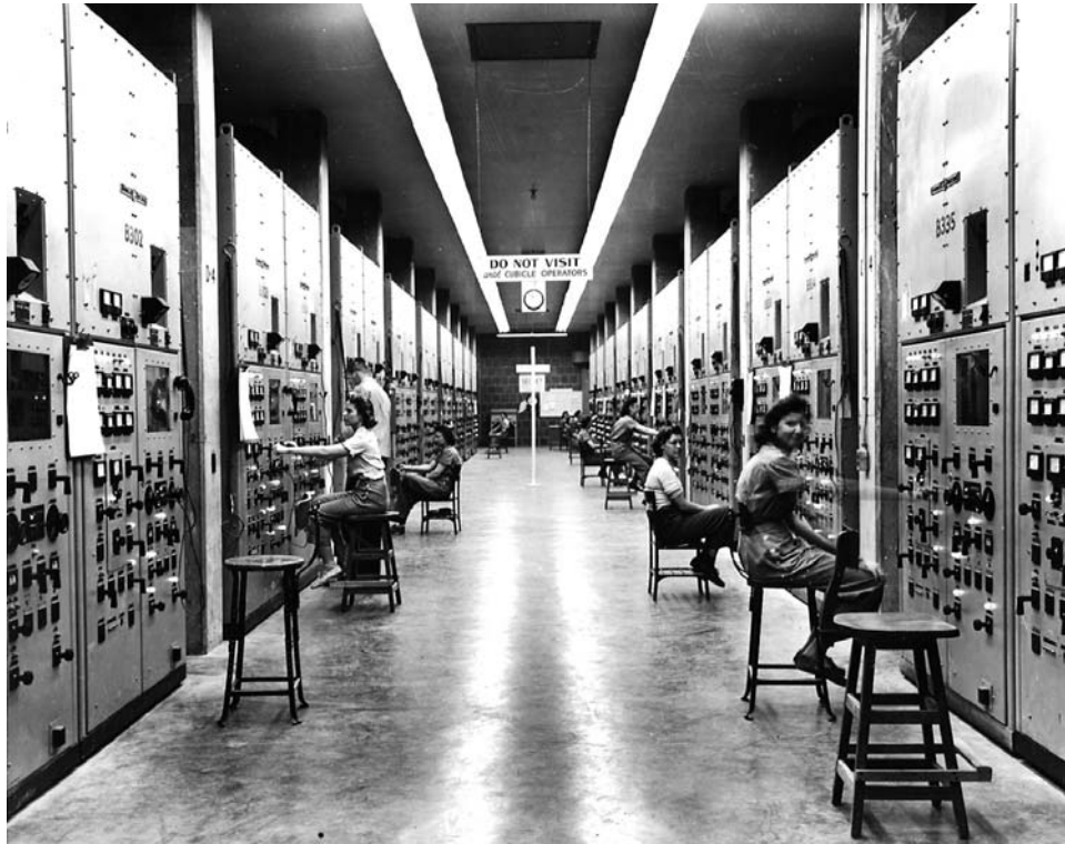
Figure 2.10 Process control cubicles for one race track (DOE)
