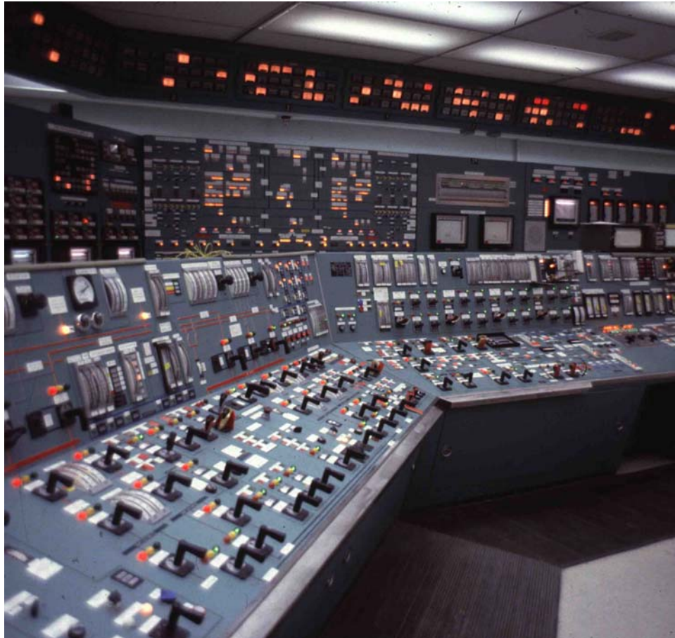
Figure 10.3 TMI Control Room
