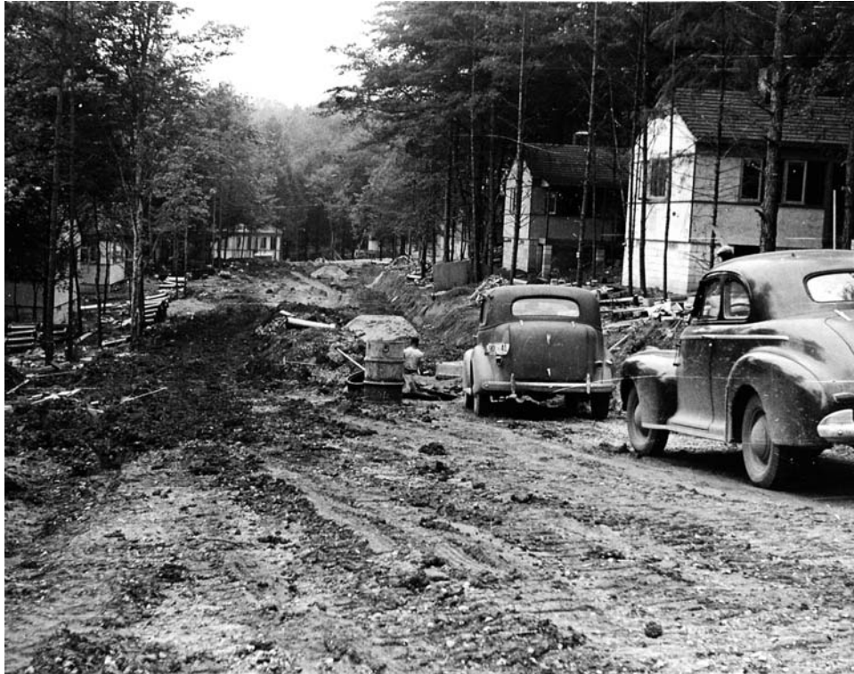
Figure 1.7 Mud presents a formidable obstacle to construction of first Oak Ridge roads and houses (DOE)
