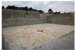
The floor of the future nuclear reactor unit, dug into the rock (300000m3 removed).
