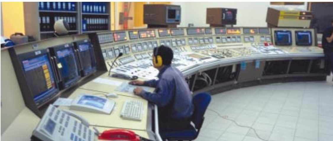
Computer system during commissioning test
