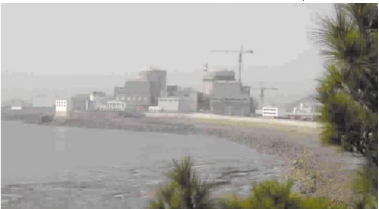
Qinshan phase 2: 2 x 600 MWe
