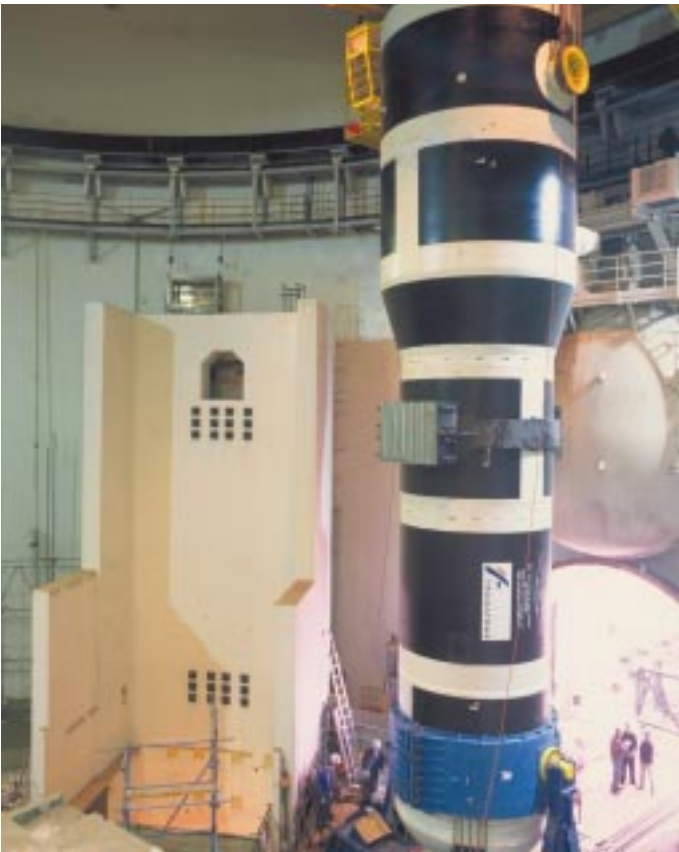
Steam generator installation
