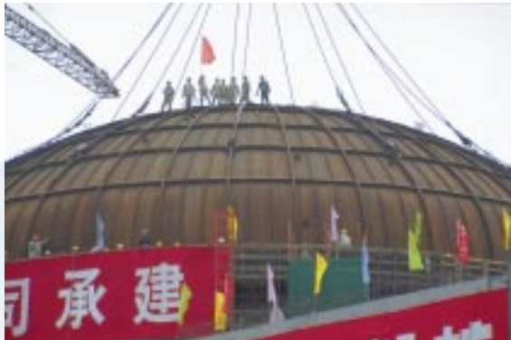
Construction of dome
