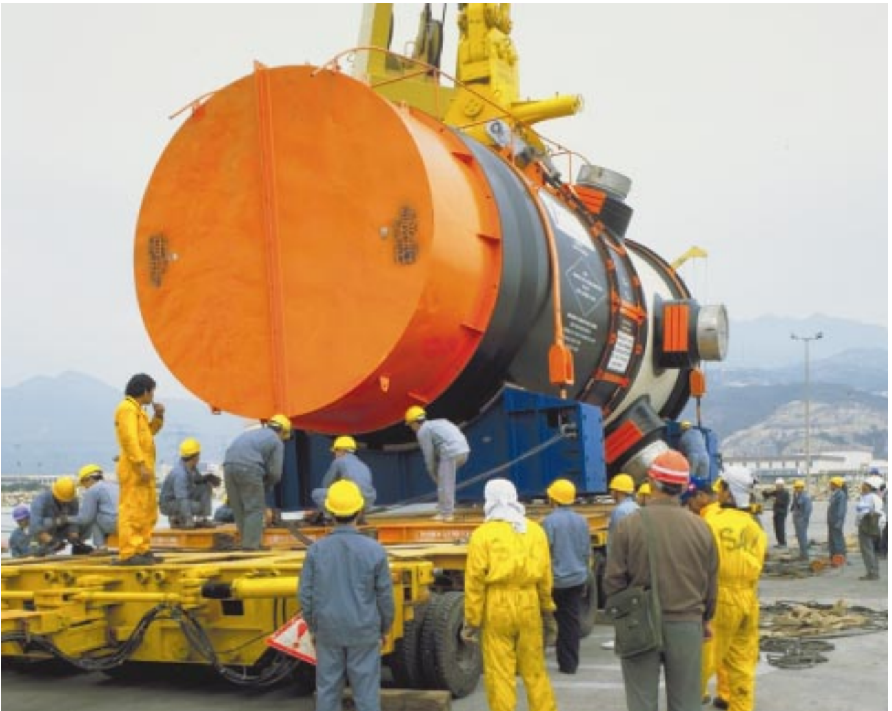
Reactor vessel handling
