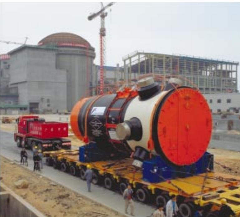
Ling Ao 1 Reactor vessel transportation
