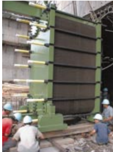
Component cooling heat exchanger
