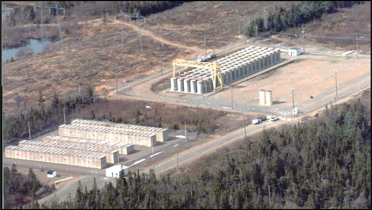
Figure 6. A Typical Spent Fuel and Radioactive Waste, Surface-Storage Facility in Canada. The Cylindrical Concrete Canisters in the Background (100 of them) are sufficient to safely hold the approximately 1000 Tonnes of Spent Fuel from about 10 Years of Full Power Operation of a CANDU Reactor. The Site will accommodate 200 more such Canisters to securely contain all Spent Fuel from at least Thirty Years of Reactor Operation. The Concrete Structures in the Foreground hold relatively low to moderate dose rate Maintenance and Process Wastes. (Photo, Courtesy of NB Power).
