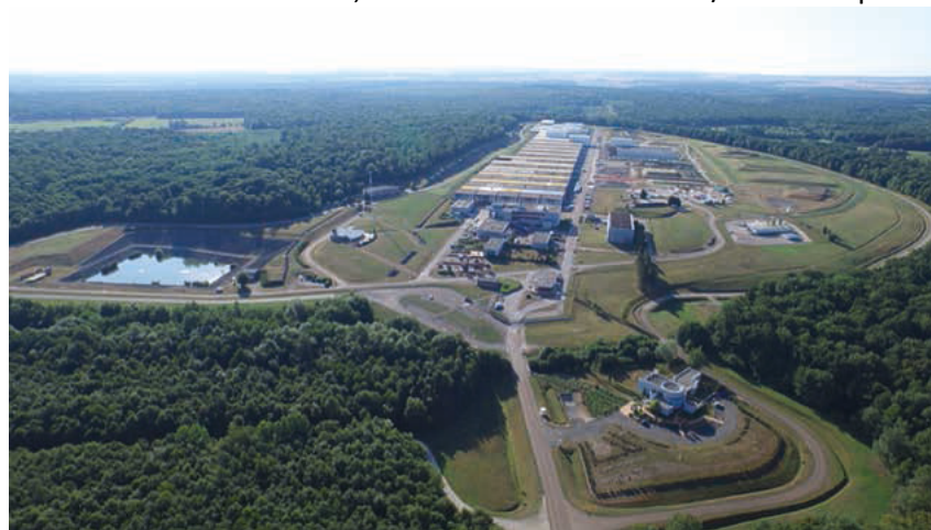
Figure 6. LILW Andra disposal, France
