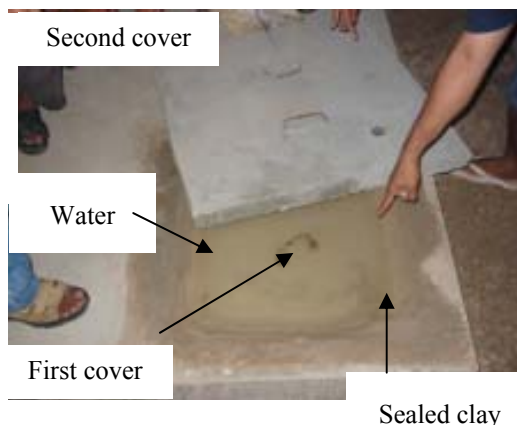
Fig 10: Technical hole and its two covers
