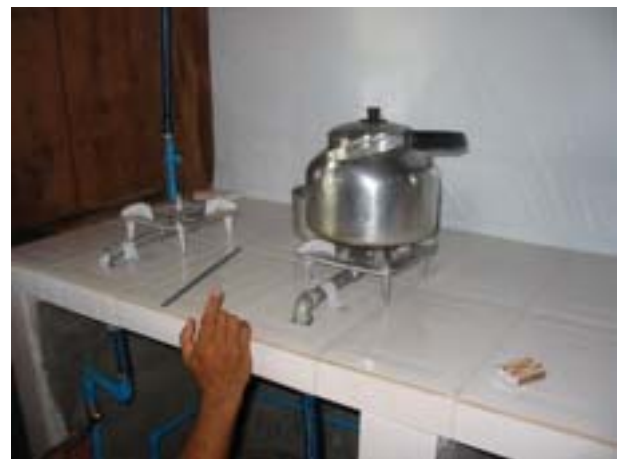
Fig 19: Installing gas burner
