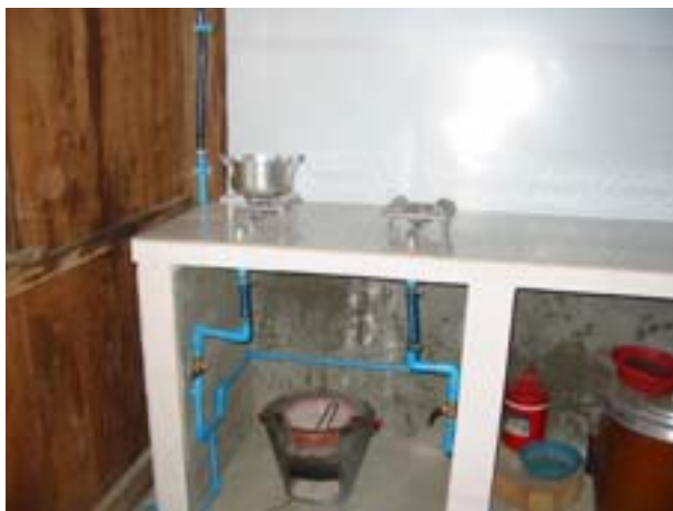
Fig 19: Installing gas burner
