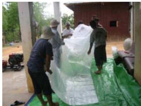
Fig 16: Assembling two plastic layers for gas reservoir
