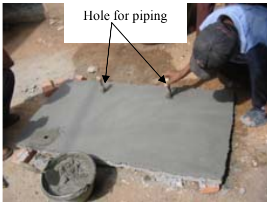
Fig 11: Plan and construction of worktop for cooking
