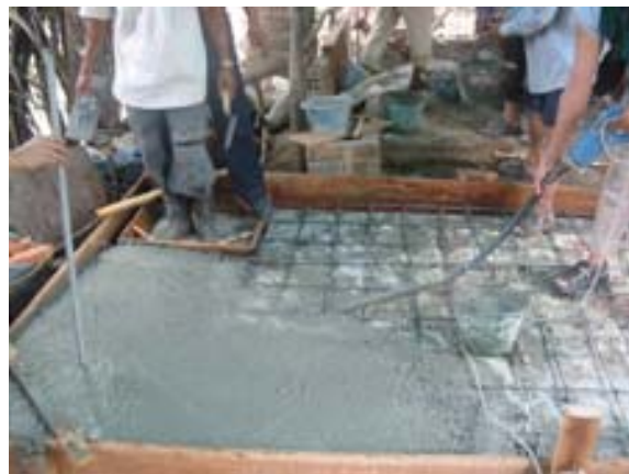
Fig 9: Vibrating concrete
