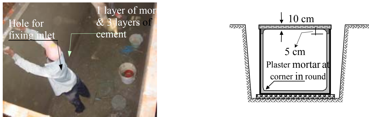
Fig 4: Plastering mortar inside the tank to protect leakage
