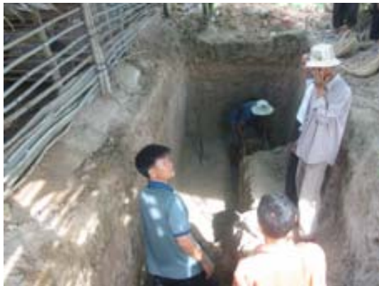
Fig 1: Digging digester hole and underground
