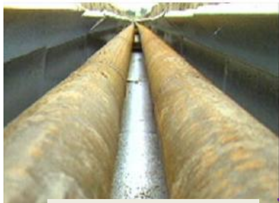
Main Transport Line
