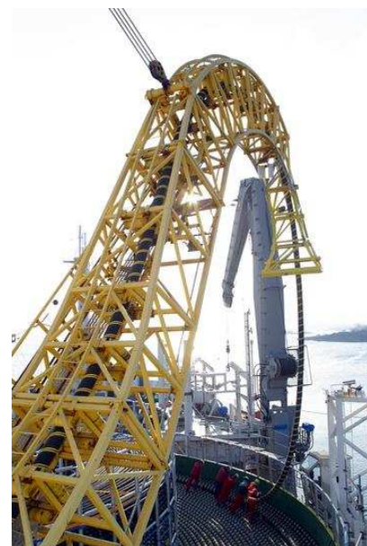
Figure 25.6. Laying a high-voltage DC link between Finland and Estonia. A pair of these cables transmit a power of 350 MW. Photo: ABB.
