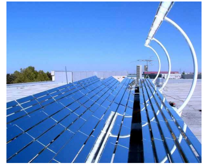
Figure 6.20. A combined-heat-and-power photovoltaic unit from Heliodynamics. A reflector area of 32 m 2 (a bit larger than the side of a double-decker bus) delivers up to 10 kW of heat and 1.5 kW of electrical power. In a sun-belt country, one of these one-ton devices could deliver about 60 kWh/d of heat and 9 kWh/d of electricity. These powers correspond to average fluxes of 80 W/m 2 of heat and 12 W/m 2 of electricity (that's per square metre of device surface); these fluxes are similar to the fluxes delivered by standard solar heating panels and solar photovoltaic panels, but Heliodynamics's concentrating design delivers power at a lower cost, because most of the material is simple flat glass.
