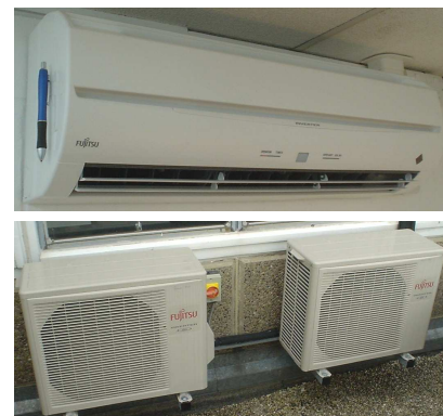
Figure 21.10. The inner and outer bits of an air-source heat pump that has a coefficient of performance of 4. The inner bit is accompanied by a ball-point pen, for scale. One of these Fujitsu units can deliver 3.6 kW of heating when using just 0.845 kW of electricity. It can also run in reverse, delivering 2.6 kW of cooling when using 0.655 kW of electricity.
