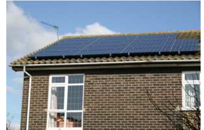
Figure 6.5. Solar photovoltaics: data from a 25-m 2 array in Cambridgeshire in 2006. The peak power delivered by this array is about 4 kW. The average, year-round, is 12 kWh per day. That's 20 W per square metre of panel.
