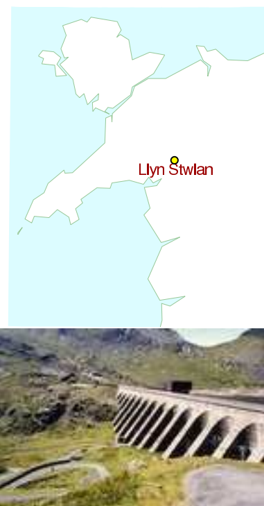
Figure 26.5. Llyn Stwlan, the upper reservoir of the Ffestiniog pumped storage scheme in north Wales. Energy stored: 1.3 GWh. Photo by Adrian Pingstone.
