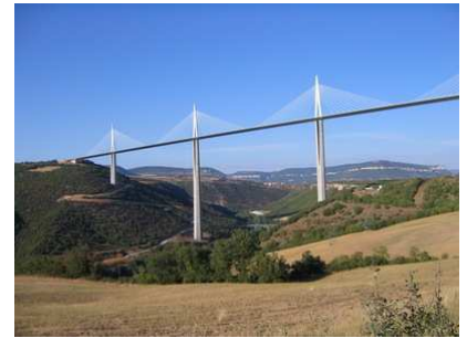
Figure H.4. Millau Viaduct in France, the highest bridge in the world. Steel and concrete, 2.5 km long and 353 m high.
