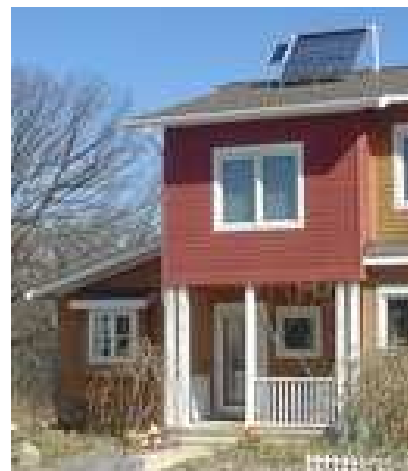
Figure 27.2. A solar water heater providing hot water for a family in Michigan. The system's pump is powered by the small photovoltaic panel on the left.
