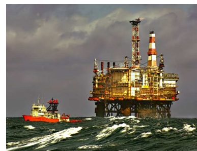
Figure 10.4. The Magnus platform in the northern UK sector of the North Sea contains 71 000 tons of steel. In the year 2000 this platform delivered 3.8 million tons of oil and gas – a power of 5 GW. The platform cost £1.1 billion.
