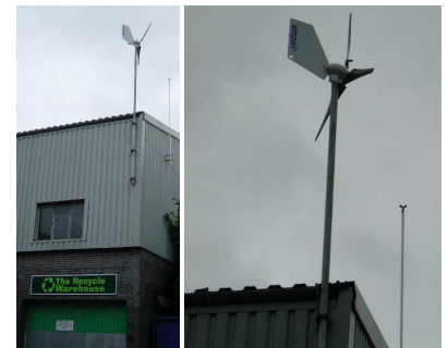
Figure B.8. An Ampair "600 W" micro-turbine. The average power generated by this micro-turbine in Leamington Spa is 0.037 kWh per day (1.5 W).
