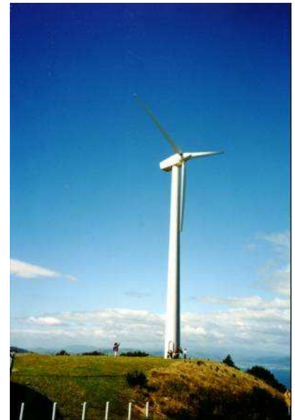
Figure B.4. The Brooklyn windmill above Wellington, New Zealand, with people providing a scale at the base. On a breezy day, this windmill was producing 60 kW, (1400 kWh per day). Photo by Philip Banks.
