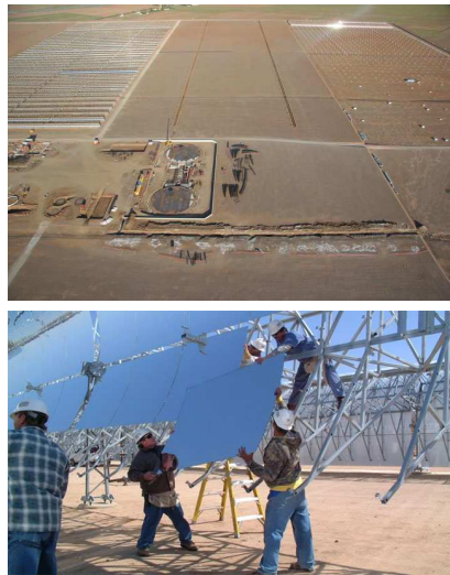
Figure 25.3. Andasol – a “100 MW” solar power station under construction in Spain. Excess thermal energy produced during the day will be stored in liquid salt tanks for up to seven hours, allowing a continuous and stable supply of electric power to the grid. The power station is predicted to produce 350 GWh per year (40 MW). The parabolic troughs occupy 400 hectares, so the power per unit area will be 10 W/m 2 . Upper photo: ABB. Lower photo: IEA SolarPACES.
