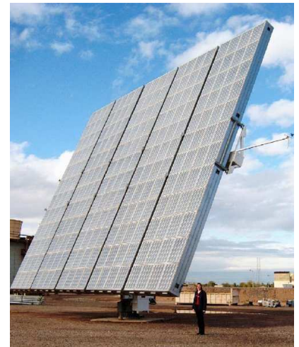
Figure 25.11. A 25 kWp concentrator photovoltaic collector produced by Californian company Amonix. Its 225 \text{ m}^2 aperture contains 5760 Fresnel lenses with optical concentration \times 260 , each of which illuminates a 25%-efficient silicon cell. One such collector, in an appropriate desert location, generates 140 kWh per day – enough to cover the energy consumption of half an American. Photograph by David Faiman.
