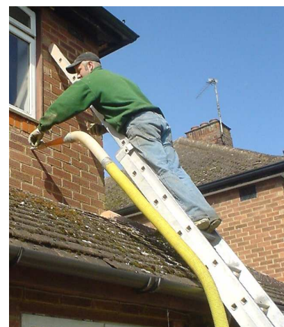
Figure 21.5. Cavity-wall insulation going in.
