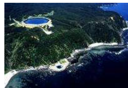
Figure 26.12. Okinawa pumped-storage power plant, whose lower reservoir is the ocean. Energy stored: 0.2 GWh. Photo by courtesy of J-Power. www.ieahydro.org .
