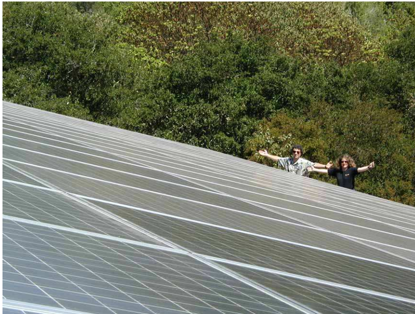
Figure 6.6. Two solar warriors enjoying their photovoltaic system, which powers their electric cars and home. The array of 120 panels (300 W each, 2.2 m 2 each) has an area of 268 m 2 , a peak output (allowing for losses in DC-to-AC conversion) of 30.5 kW, and an average output – in California, near Santa Cruz – of 5 kW (19 W/m 2 ). Photo kindly provided by Kenneth Adelman.
