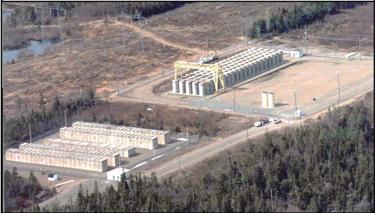
Figure 6. A Typical Spent Fuel and Radioactive Waste, Surface-Storage Facility in Canada. The Cylindrical Concrete Canisters in the Background (100 of them) are sufficient to safely hold the approximately 1000 Tonnes of Spent Fuel from about 10 Years of Full Power Operation of a CANDU Reactor. The Site will accommodate 200 more such Canisters to securely contain all Spent Fuel from at least Thirty Years of Reactor Operation. The Concrete Structures in the Foreground hold relatively low activity Maintenance and Process Wastes. (Photo, Courtesy of NB Power).
